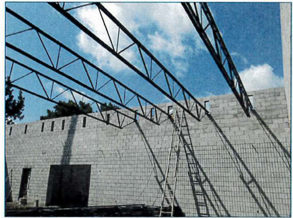
St. Kateri Tekakwitha Catholic Church, Dearborn, MI Addition/Renovation
