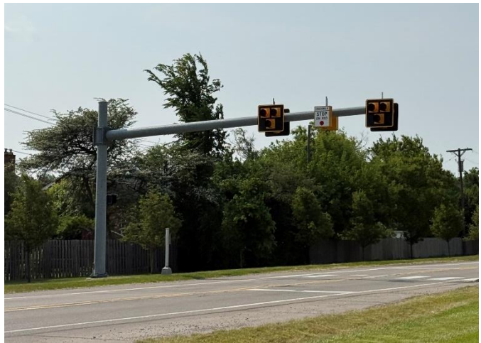
HAWK Signal near Sydney Blvd and Park St provides a mid-block pedestrian crosswalk.
