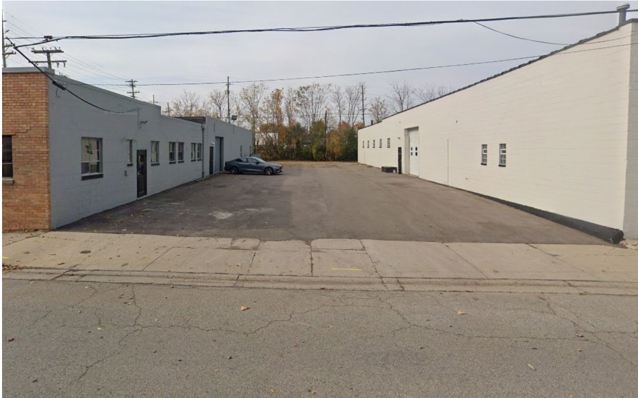
Figure 2. Streetview of Existing Parking Lot Between Buildings Abutting Amelia
