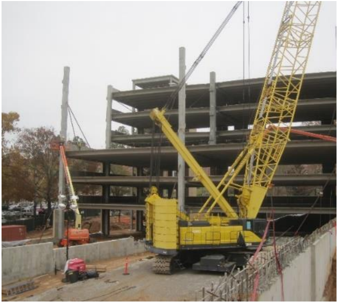
Photo 2 – Crane used for precast erection, and partially erected precast parking structure.
