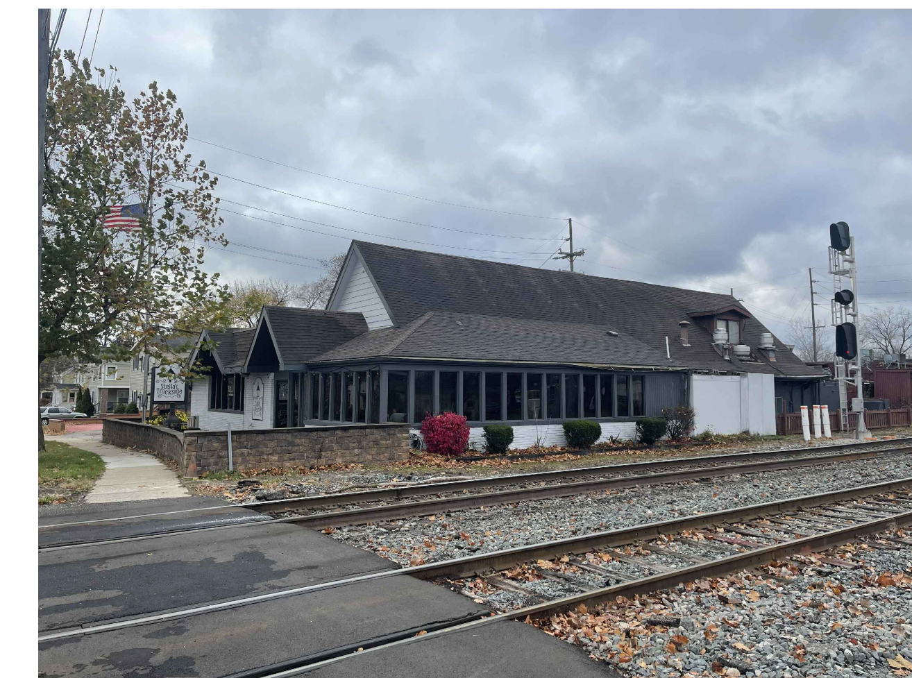
EXISTING LOOKING SOUTHWEST
