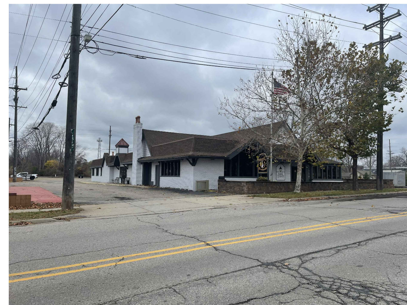
EXISTING LOOKING NORTHWEST
