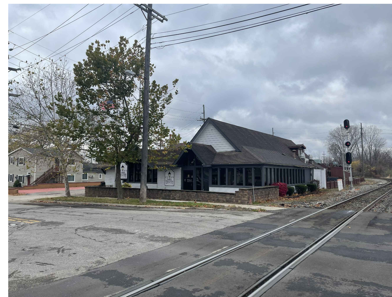
EXISTING LOOKING WEST
