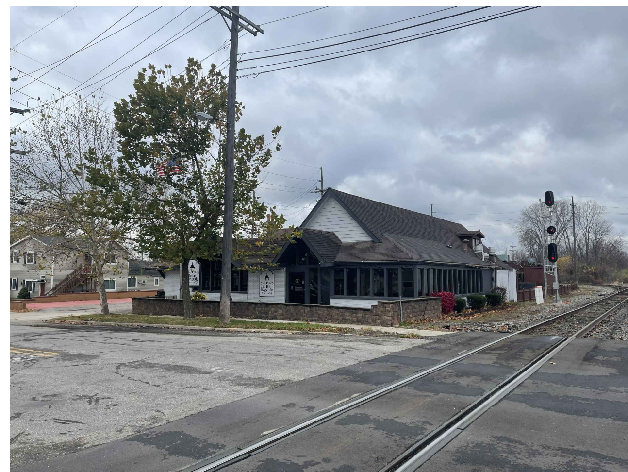
EXISTING LOOKING WEST
