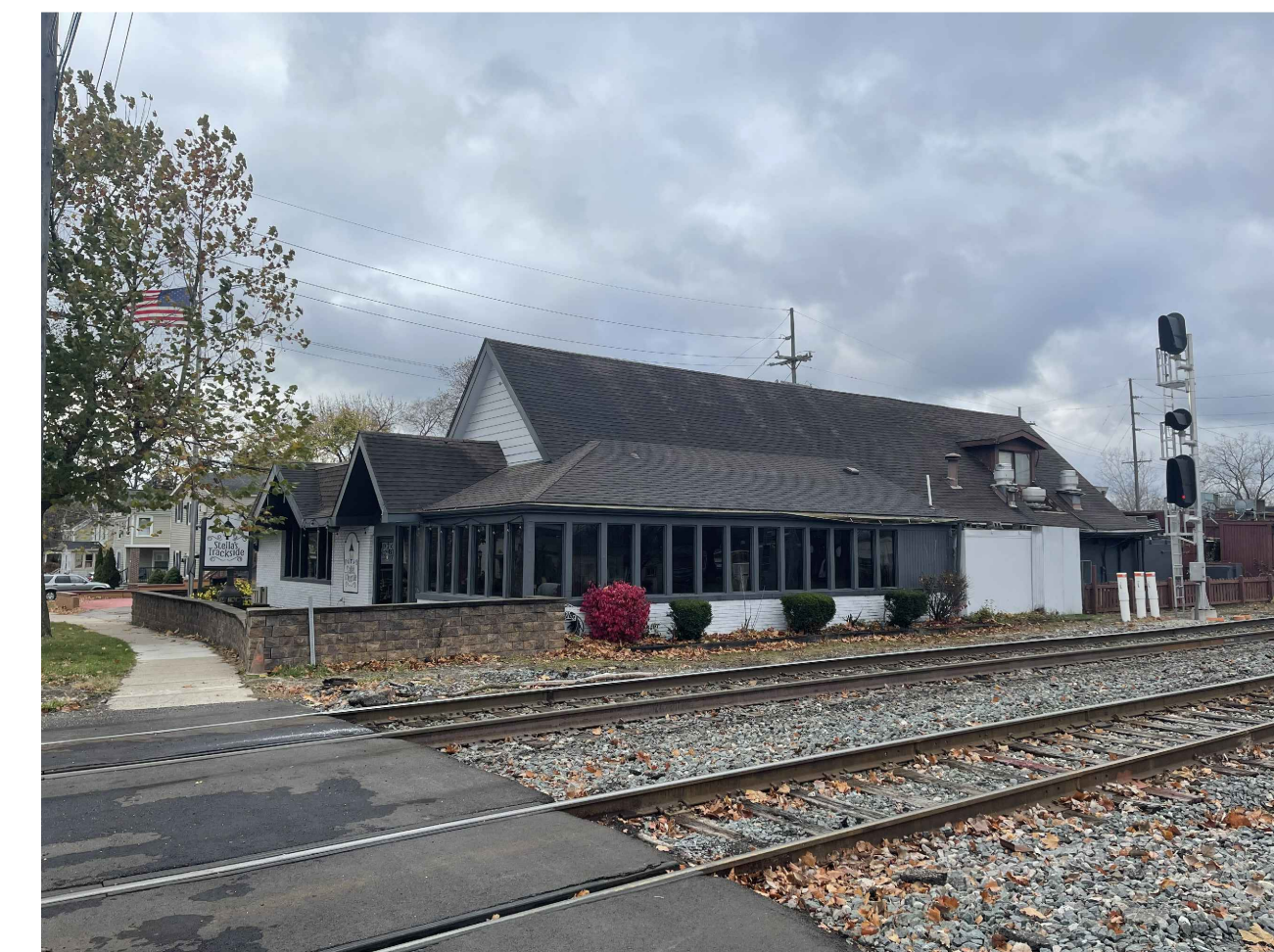
EXISTING LOOKING SOUTHWEST
