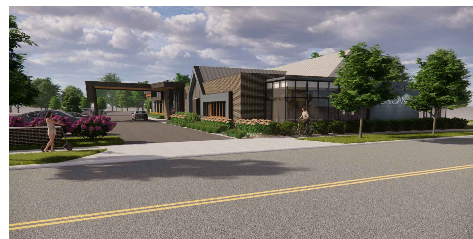
EXISTING LOOKING NORTHWEST
