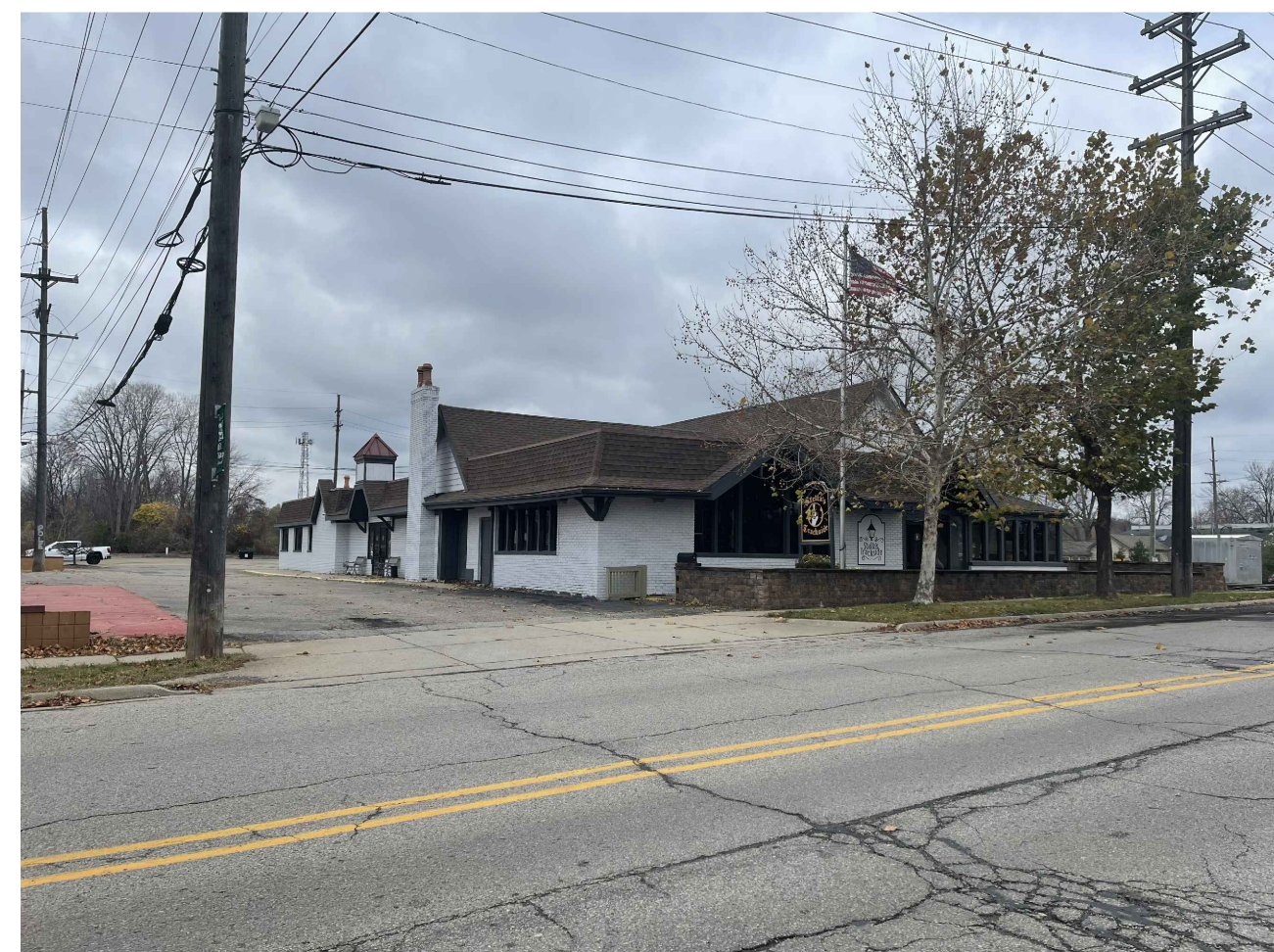
EXISTING LOOKING NORTHWEST
