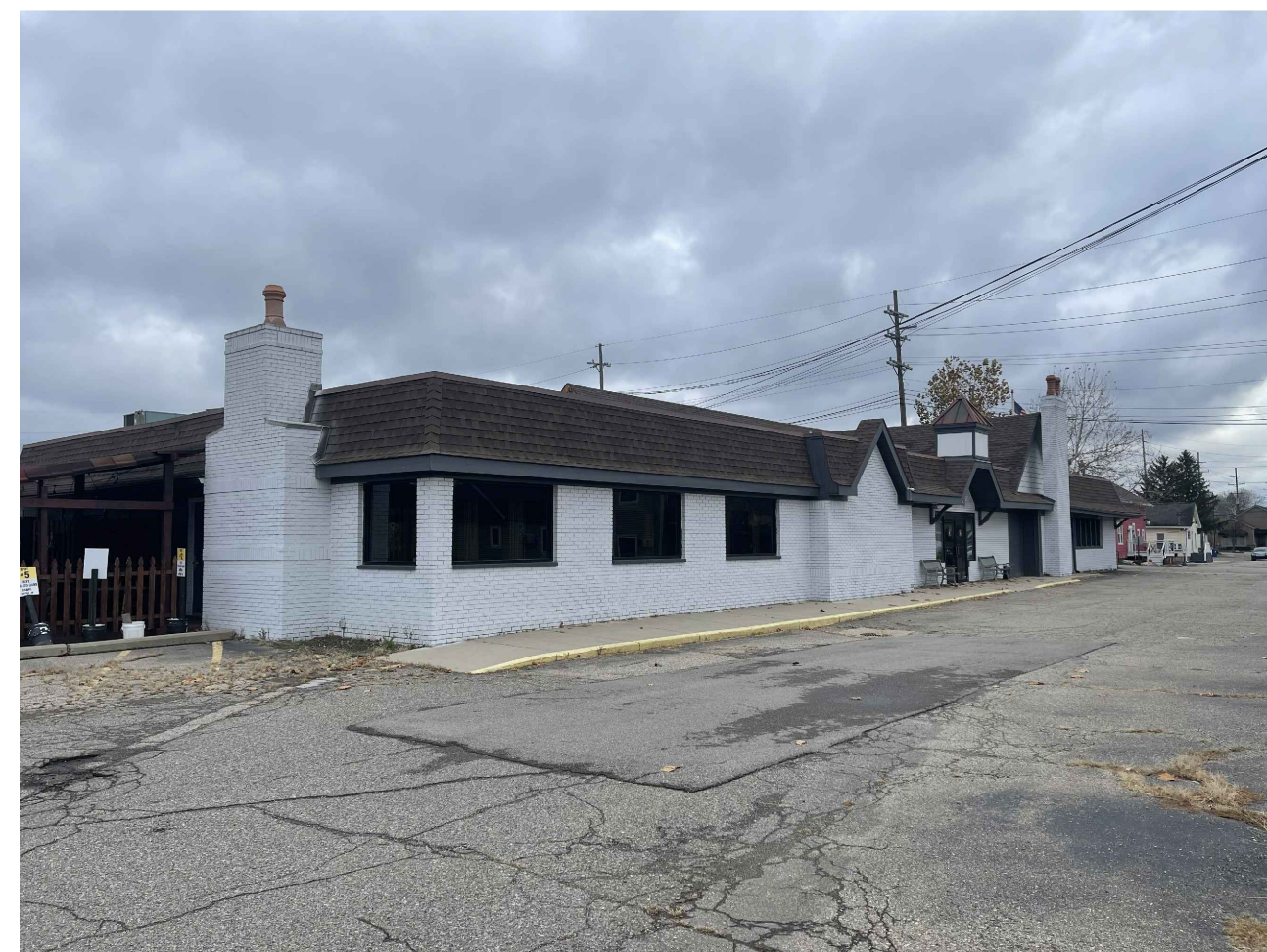
EXISTING LOOKING NORTHEAST
