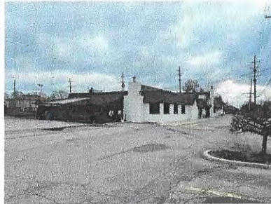
EXISTING LOOKING NORTHEAST IMAGE NUMBER E-6.0
