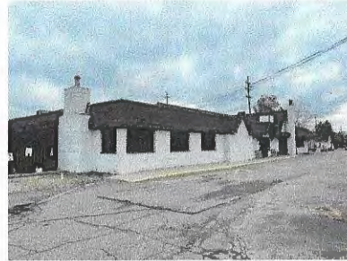
EXISTING LOOKING NORTHEAST IMAGE NUMBER E-5.0
