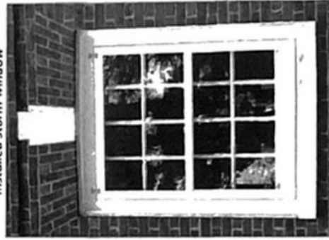
Installed storm window
